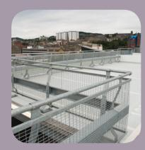
Part 1 1996. With a zero footprint in the parking bay, Brisafe allows architects to maximise the parking space available, while providing a flexible system that 'gives' on impact to minimise damage to vehicles and the barrier itself.
