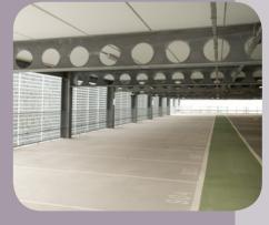
barriers floor mounted on RB1X spring steel buffers. The split level decks and pedestrian walkways were contained by Berry Beam safety barriers floor mounted on RB1 Spring steel buffers.
