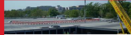
CAR PARK CONSTRUCTION & SAFETY
